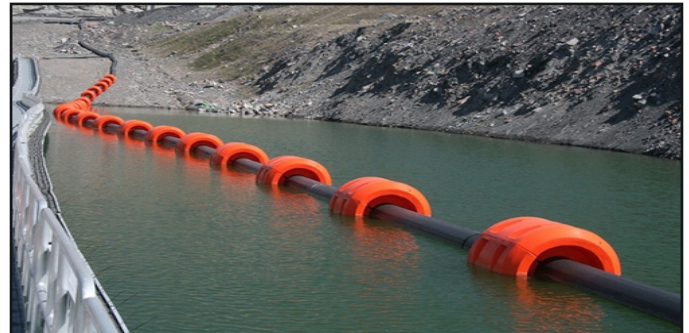
Hanging / Floating - Pipe Line
