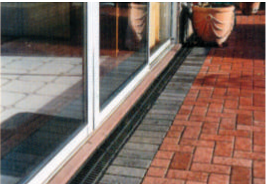
Always backfill with concrete with the grating fitted Haunch concrete up and around channel without leaving any empty spaces
